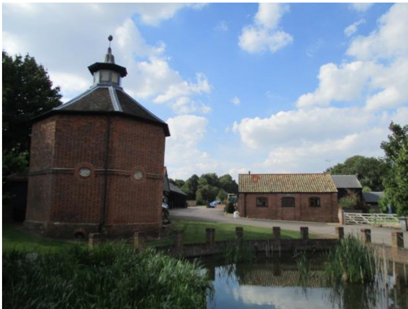
Dovecote at Manor Farm. circa 1700 Grade II*
